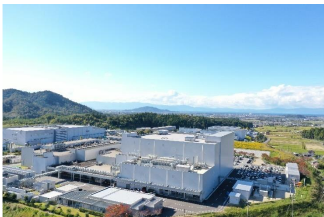
Shiga PSC Third Building (Center)
