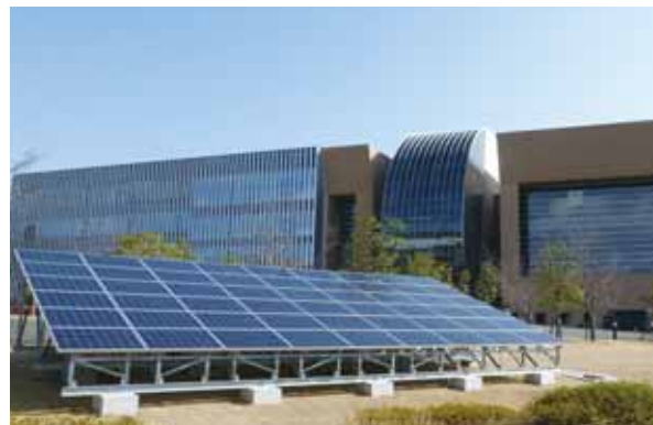
A solar power generation system at the Nara Research and Development Center
