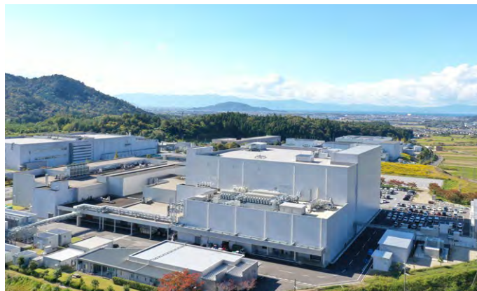
Shiga Product Supply Center (new building shown in the center)
