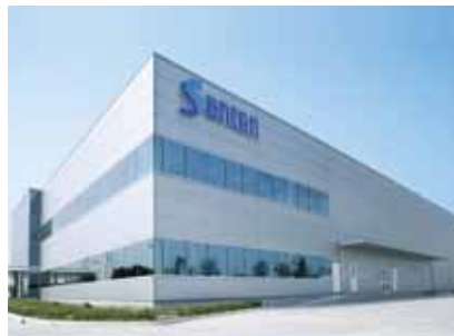
④ Suzhou Plant (China)
